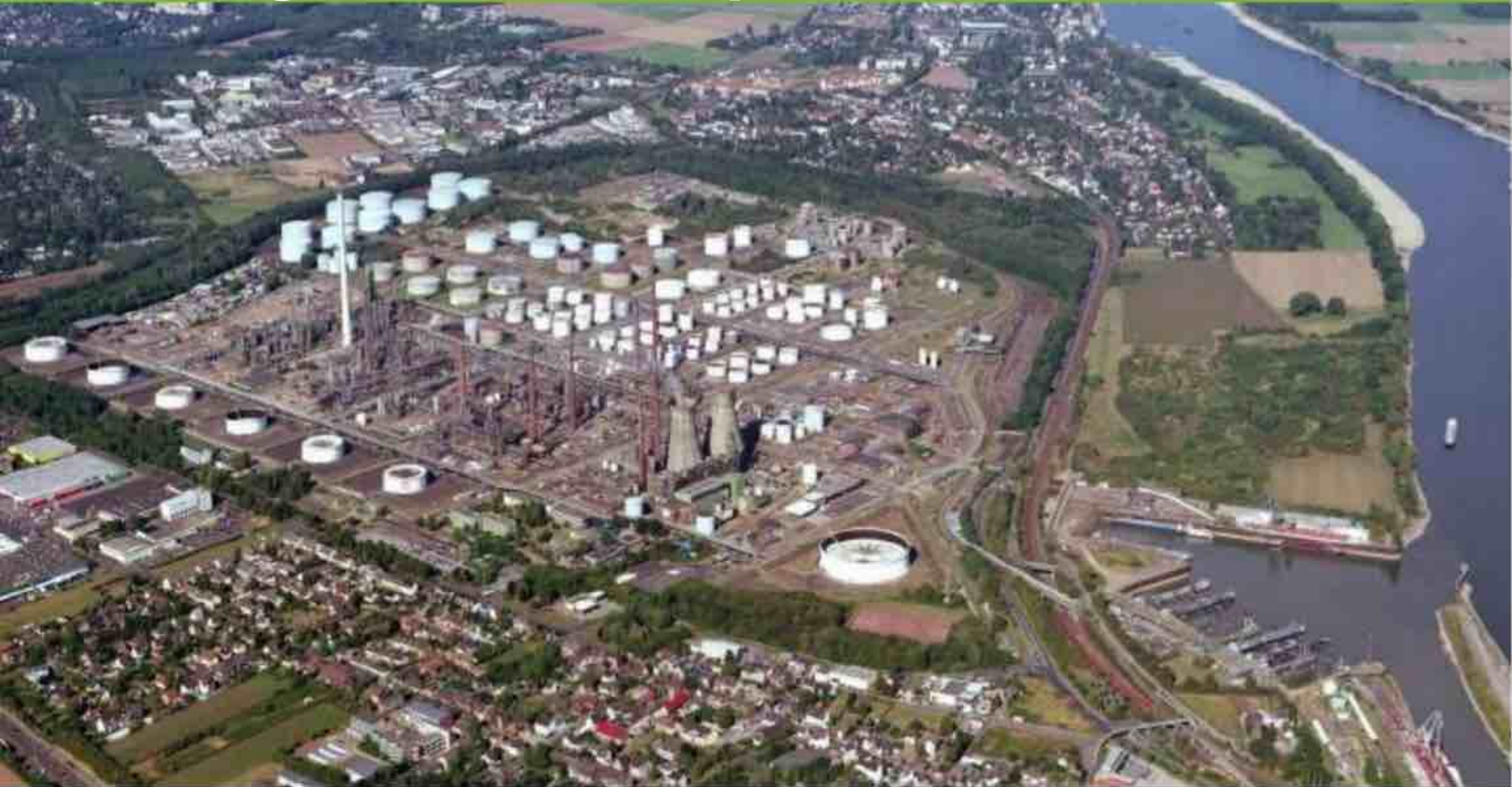
Shell Godorf refineries – Cologne Germany
