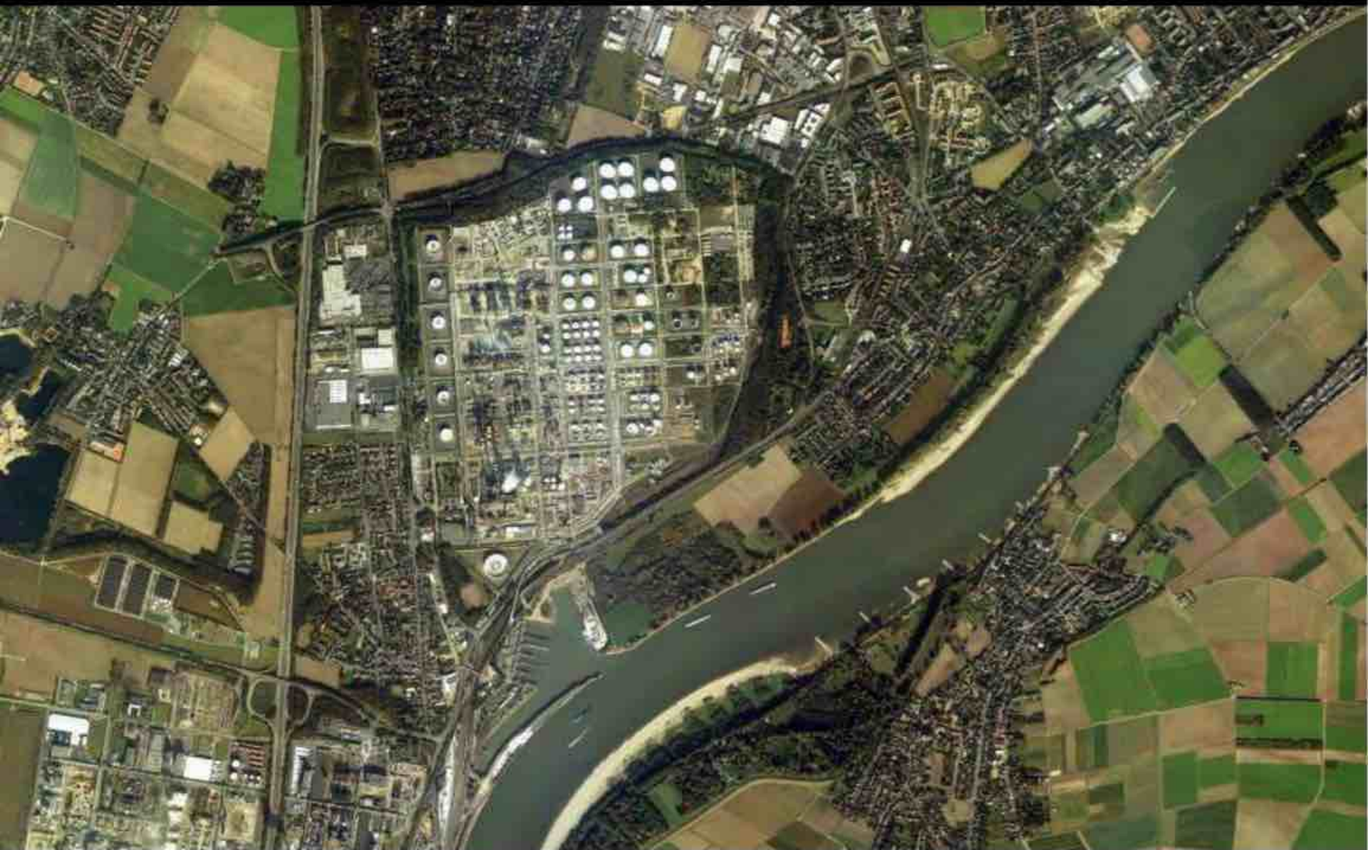
Shell Godorf refineries – Cologne Germany
