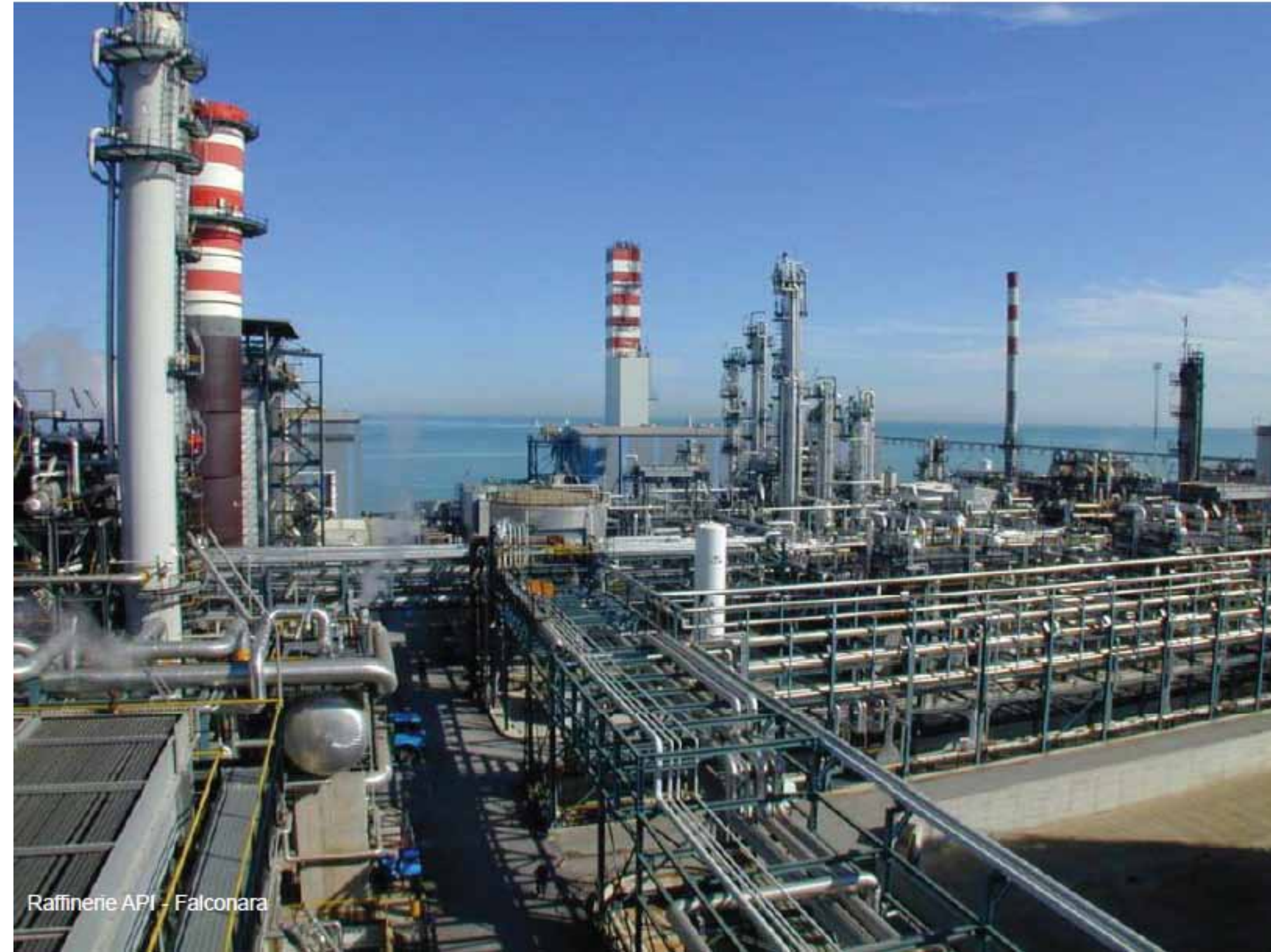
Raffinerie API, Falconara, Ancona
